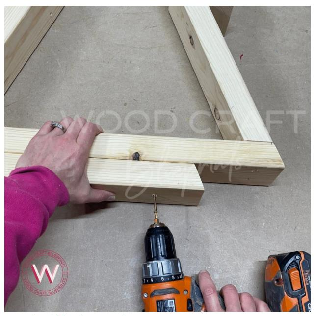
Fasten "trunk" from bottom with 2 screws.
